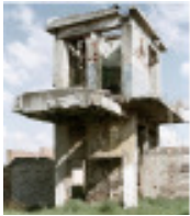
The Docrats' lavatory, Fietas, Johannesburg, 17 March 2003.
